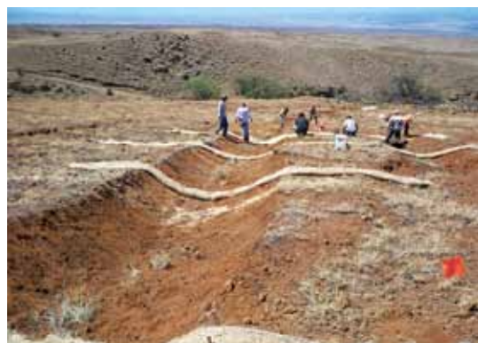
Figure 55: Project staff installing erosion control fabric in the watershed. Photo credit: Kohala Watershed Partnership
